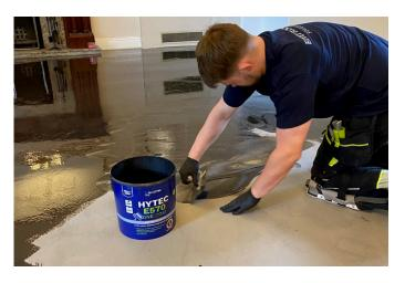
Capable of suppressing residual construction moisture in cementitious subfloors up to 99% RH, it provided reliable, long-term moisture protection for the floor covering system.
