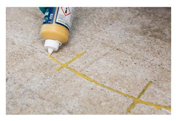
areas, the Bostik team advised that Blade Flooring apply its HYTEC E570 ONE COAT damp-proof membrane (DPM) to suppress the residual moisture in the subfloor, followed by GRIP A526 UNIVERSAL PRIMER and SCREEDMASTER SL C540 FLOW smoothing compound, which provides improved workability and excellent flow characteristics.
